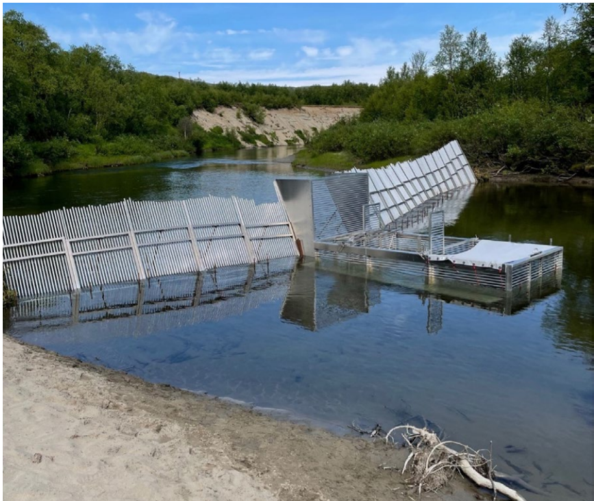
Figure 3. Picket weir in the river Máskejohka, a tributary to the Tana. Photo: Eirik Frøiland
