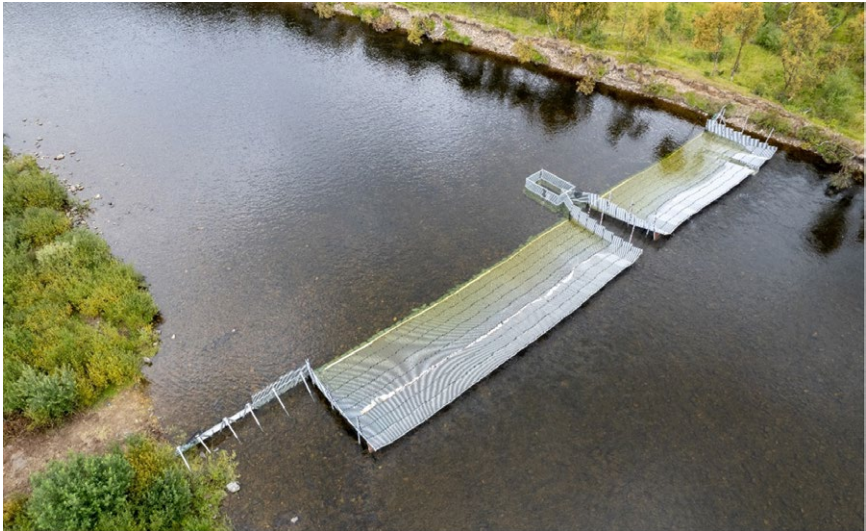
Figure 4. Resistance board weir in the river Vestre Jakobselv. Photo: Jan Harald Tomassen
